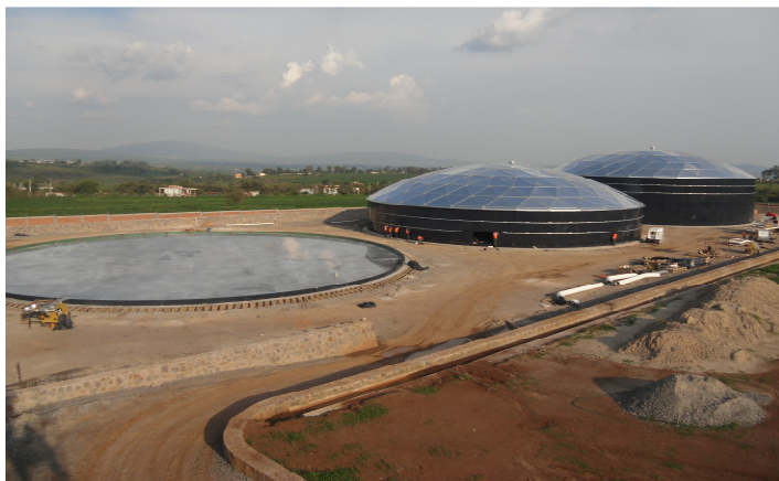
Serbatoi acqua potabile
