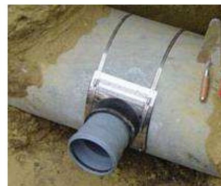
T-flex application on PVC or HDPE pipe
