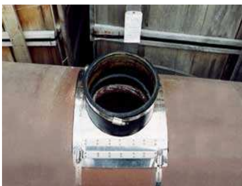
T-flex application on clay pipe
