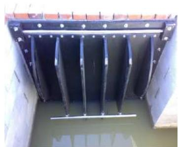
Clapet in PVC in-line conleva
