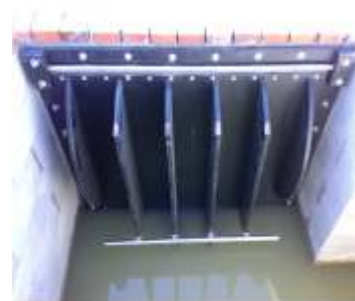
Clapet in polietilene "HDPE-S" flap valve
