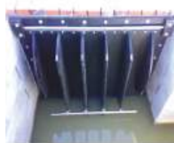
Clapet in polietilene "HDPE-S" flap valve
